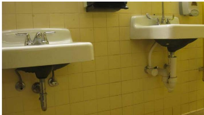
Photo 13 – Exposed pipes can pose a burning hazard
