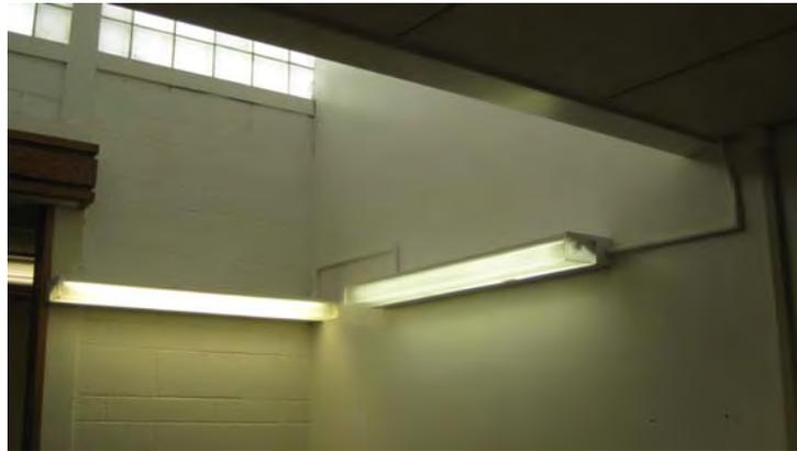
Photo 7 – Insufficient infrastructure and CMU wall construction has resulted in unsightly wiring around most classrooms
