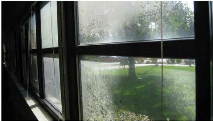
Photo 16A – Hazing of windows as glazing seals allows water migration between glazing
