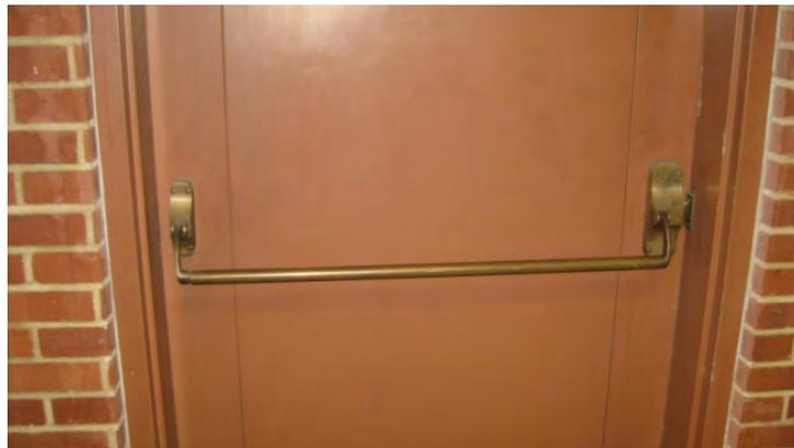
Photo 18B – Original panic hardware does not meet force limitations for accessibility requirements
