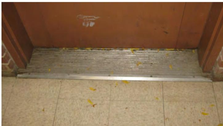
Photo 3 – Accumulation of debris/water damage at sill
