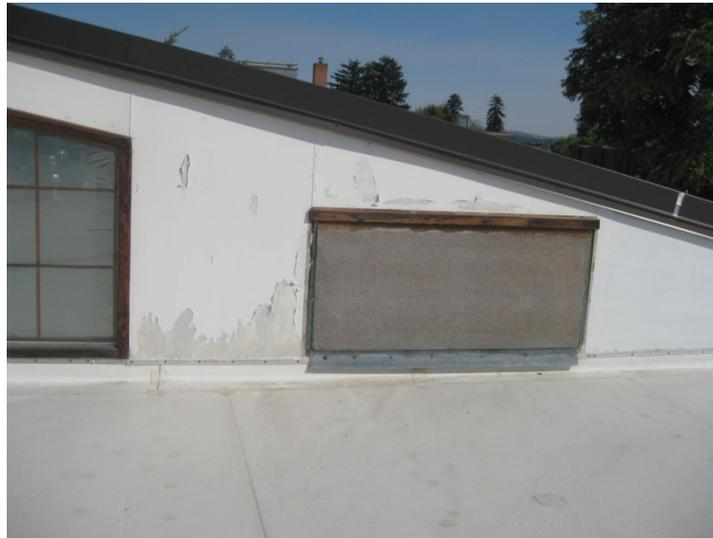
Photo 11 – Paint is peeling at roof panels; caulking is reaching the end of its life span
