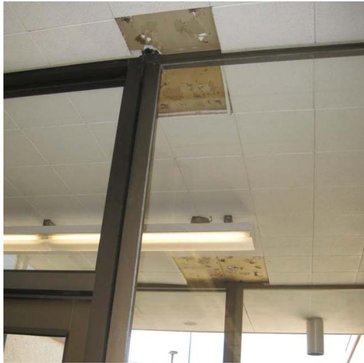
Photo 9 – Ceiling tiles adhesive is failing
