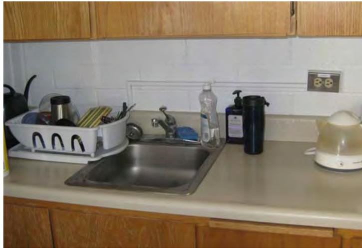
Photo 14 – Lack of GFCI outlet adjacent to water source
