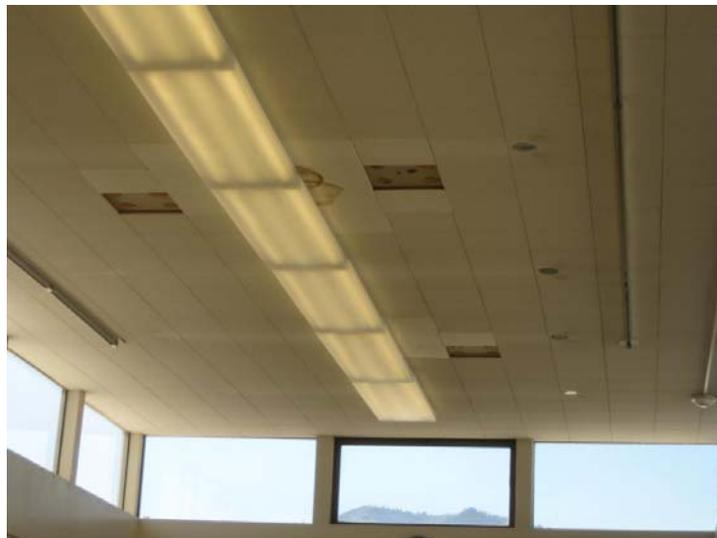
Photo 8 – Water damaged/missing ceiling tiles
