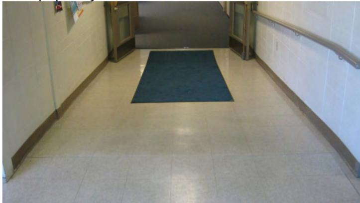
Photo 17A – Ramp in corridor (along egress path) lacks level surface prior to placement of doors
