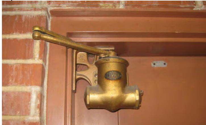
Photo 18A – Original door closers do not meet force limitations for accessibility requirements
