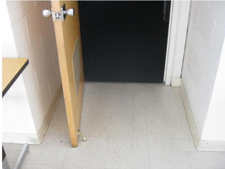
Photo 1 – Door does not have adequate accessibility clearance
