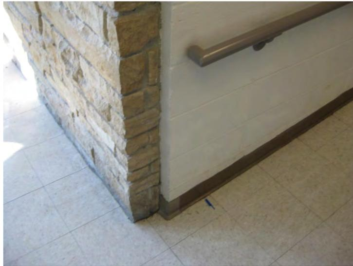
Photo 17B – Location of handrail relative to bottom of ramp does not meet egress requirements
