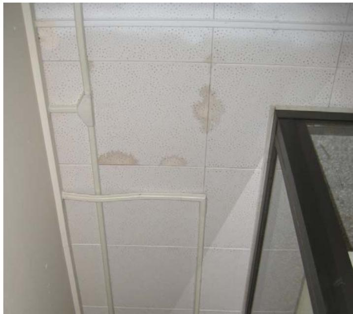
Photo 6 – Evidence of water damage on ceiling tiles and surface mounted electrical as the result of inflexible building systems
