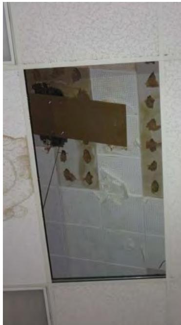
Photo 11 – Original tiles posed a safety hazard as they fall and displace the ceiling below
