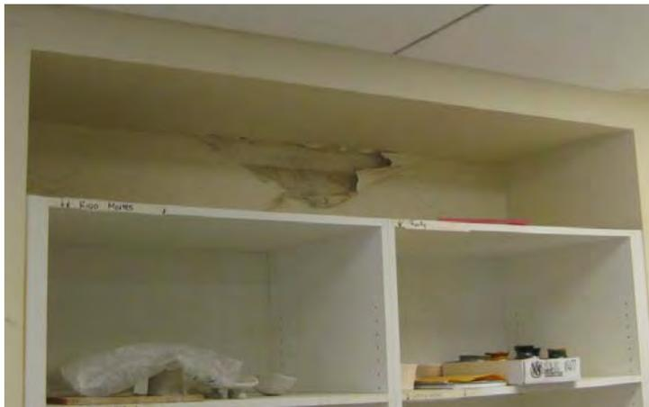
Photo 15A – Peeling paint as a result of water damage
